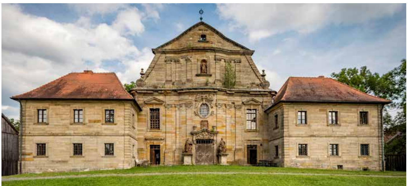
West facade of the former St. Barbara Pilgrimage Church
